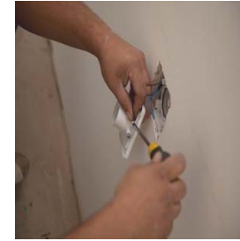
Connecting the cable to the inlet valve
