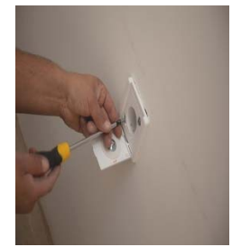
Tightening the screws to secure inlet valve
