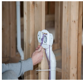
Low voltage tails secured
