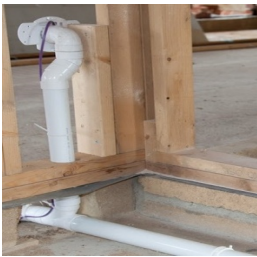
A noggin used to fix mounting box securely
