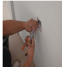
Stripping the cables
