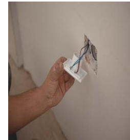
Inlet valve ready for fitting to the back box
